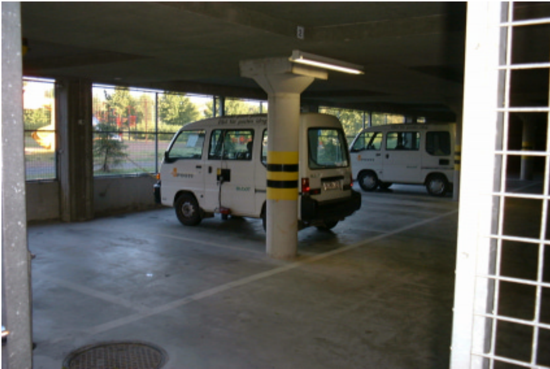
Figure 6: The electric vehicle charging facility in Raisio
