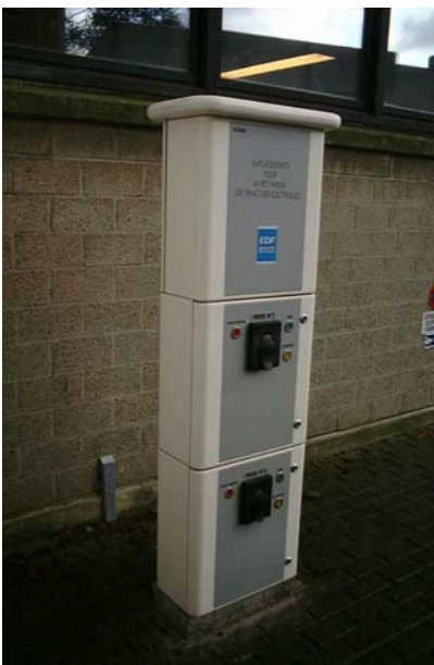
Figure 1: French –type public charging station with two outlets. The control panel and chipcard reader are at the rear; the station can control additional outlets.
