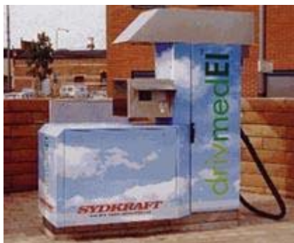
Figure 3: Fast charging station
