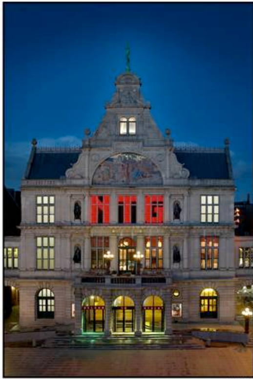
Picture 1 : The “Dutch Theatre” building illuminated consistent with the Ghent light master plan
